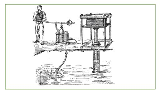
Bramah was a prolific inventor, but is patent for the hydraulic press was his most important patent. In it he descibes a hydraulic press with two cylinders and pistons of differing cross-sectional areas which is used for "obtaining and applying motive power".
